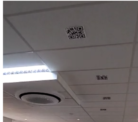
Figure 2: QR codes placed on the laboratory ceiling.
