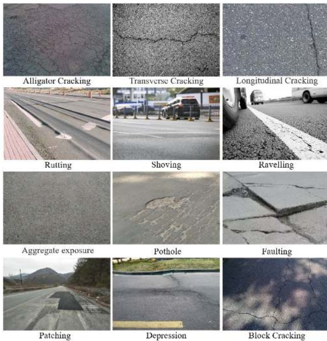
Fig. 1. Defects in Asphalt Pavement, adapted from [3].
